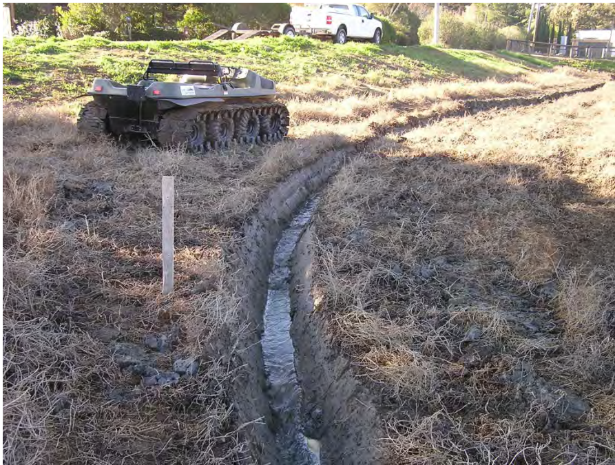
Photo 4. View newly created small circulation channel and Argo used for site access/equipment transport.
