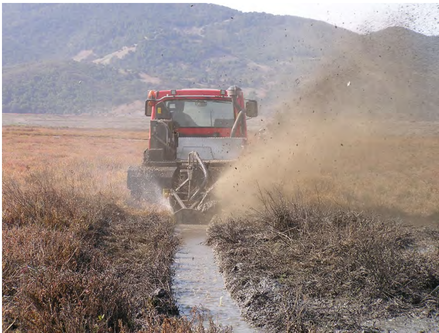
Photo 2. Ditch excavation by a mechanical rotary ditcher.
