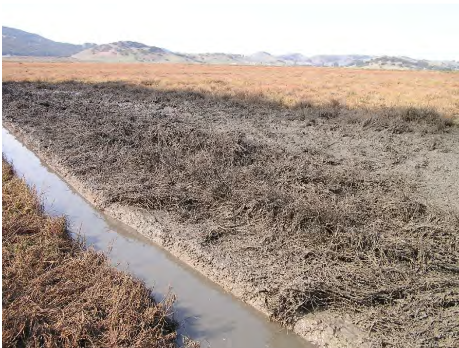
Photo 3. Image showing the circulation channel and adjacent area immediately post mechanical excavation.
