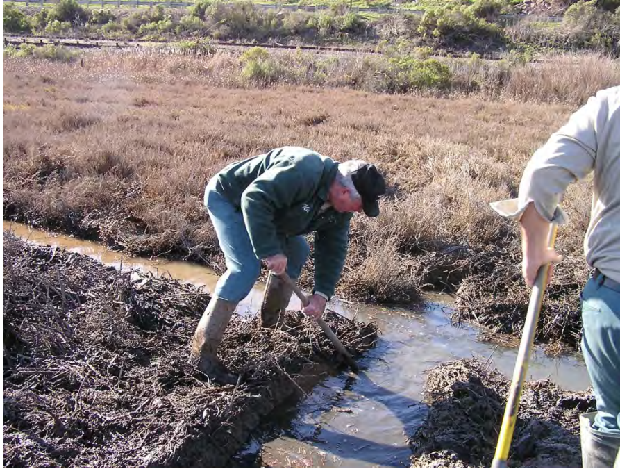
Photo 1. Ditch excavation by MAD working using hand tools.
