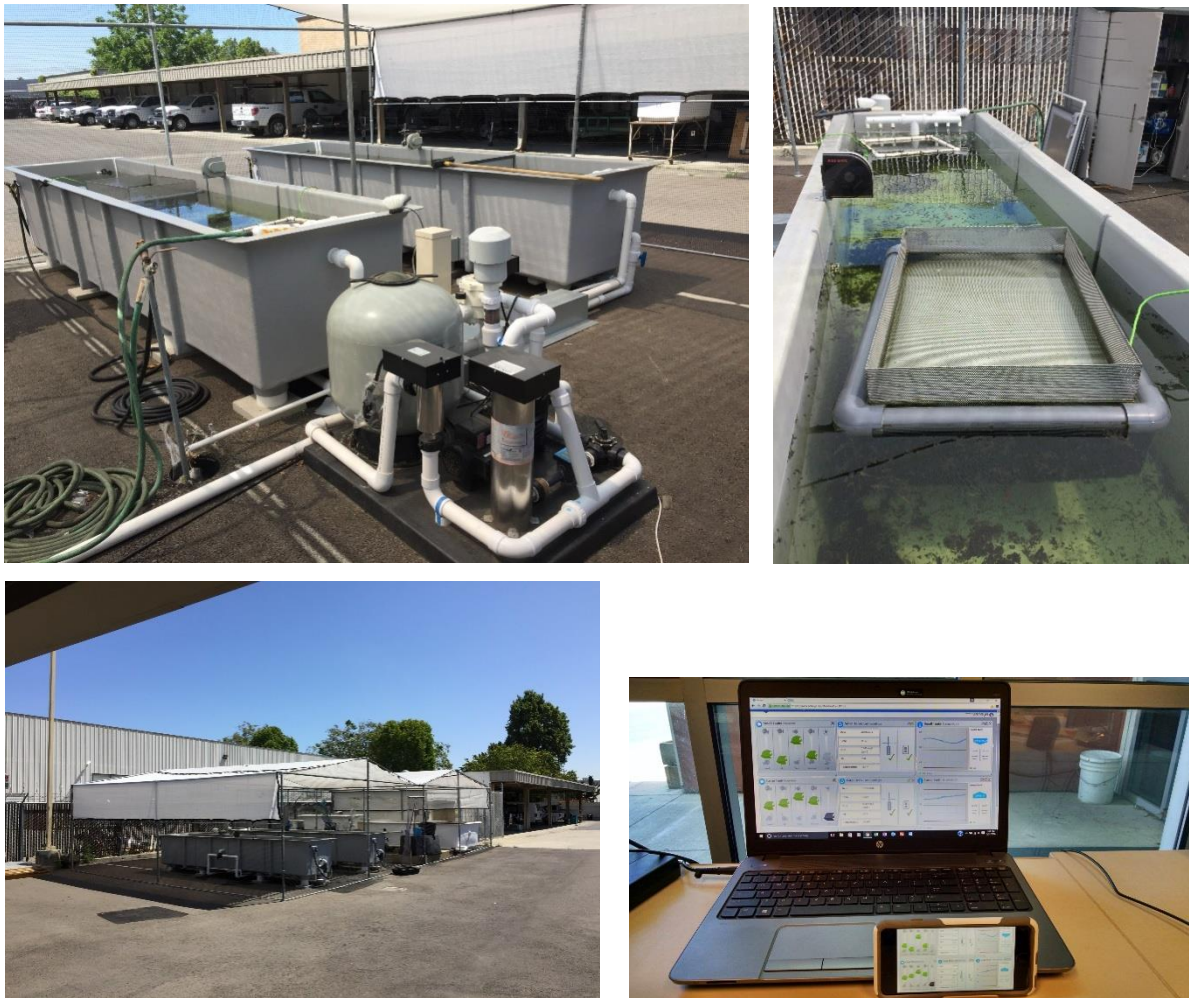
Figure 6. Two new fish tanks with pump system (top left) and fish fry tray in the tank (top right). Protective shade cloth and netting added to the tank system (bottom left). Water quality monitoring software displays (bottom right).
