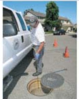
Treating storm drains
